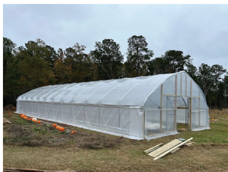
Completed high tunnel in Awendaw, SC.
