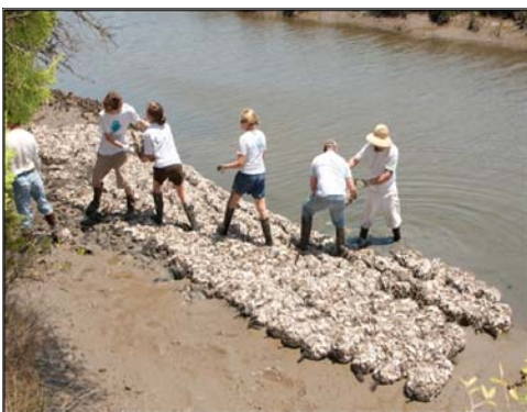
Left, Volunteers installing oyster shell at Tibwin Reef. Over 90 volunteer hours and 315 bags of shell have been used so far in restoring the reef. Photo courtesy of The Nature Conservancy. Photo taken by Keith and Sue McKeith.
