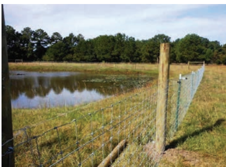
Fencing installed to protect water quality
