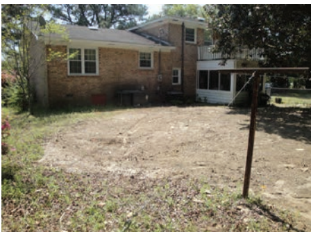
Completed Ultra Shallow Septic System Site
