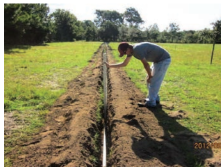
Animal Operations Project—Pipe Installation Shawn Stormer, NRCS, inspects pipe line
