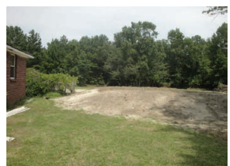
Completed Elevated Septic Installation
