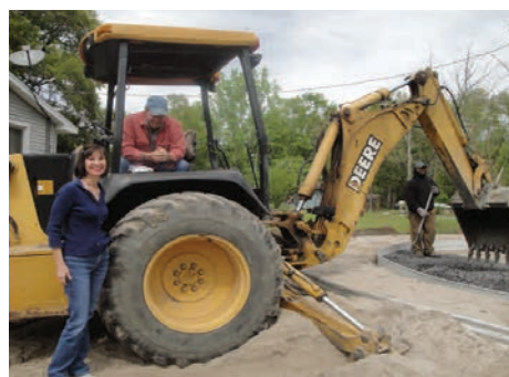
Construction site—Elevated Septic Installation Debbie Eckard shown with Septic Contractor Harry Wilson of A-1 Septic Services
