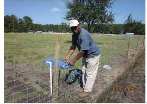
Animal Operations Project—Herman White of White's Construction install fence
