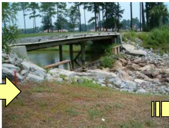
Spill way over rip rap to
