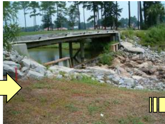
Spill way over rip rap to
