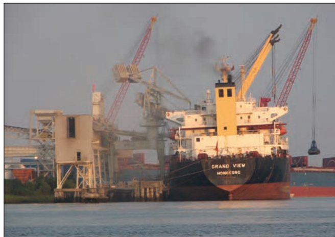
Bulk handling facilities on the Cooper River in Charleston, SC.
