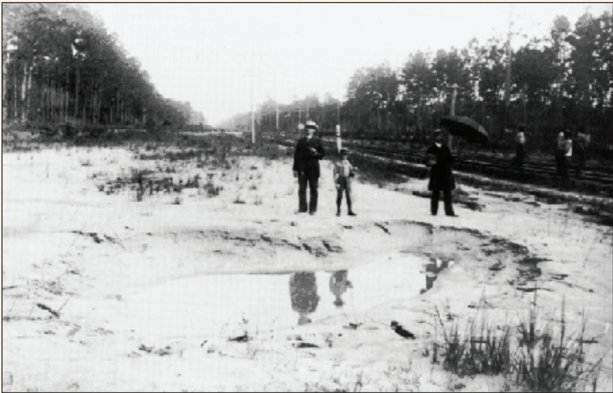
An example of a sand blow, generally referred to as liquefaction, associated with the Charleston 1886 Earthquake.
