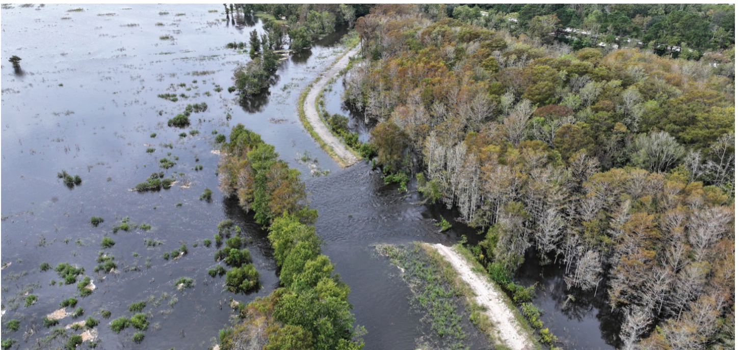
FIGURE 9. A perimeter dike breach on Santee Delta East WMA. This damage occurred from extensive flooding associated with Hurricane Helene, October 2025. The breach was repaired by SCDNR staff prior to the beginning of waterfowl season, 2024-2025.
