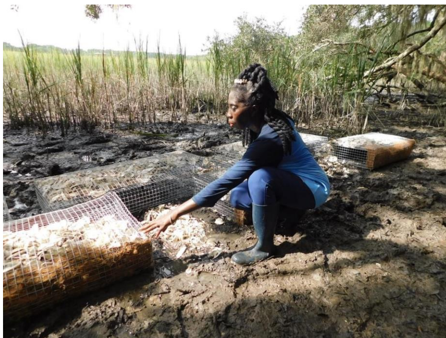
Queen Quet places manufactured wired reefs (MWRs) on the shoreline. These MWRs were created by the Gullah/Geechee Fishing Association. Photo by Kwame Sha from Gullah/Geechee Alkebulan Archive.
