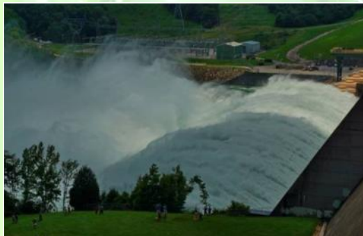
Hartwell Dam, July 9, 2013. Photo Credit: Doug Young
