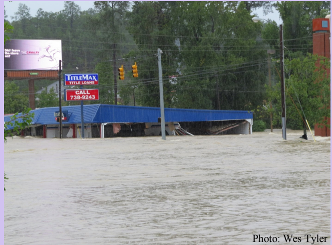
Title Max Bldg. Collapse on Garners Ferry Rd.
