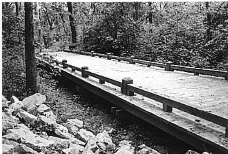
Typical wood bridge/boardwalk segment
