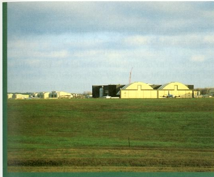
Donaldson Center Industrial Air Park began in World War II as the Greenville Army Air Base
